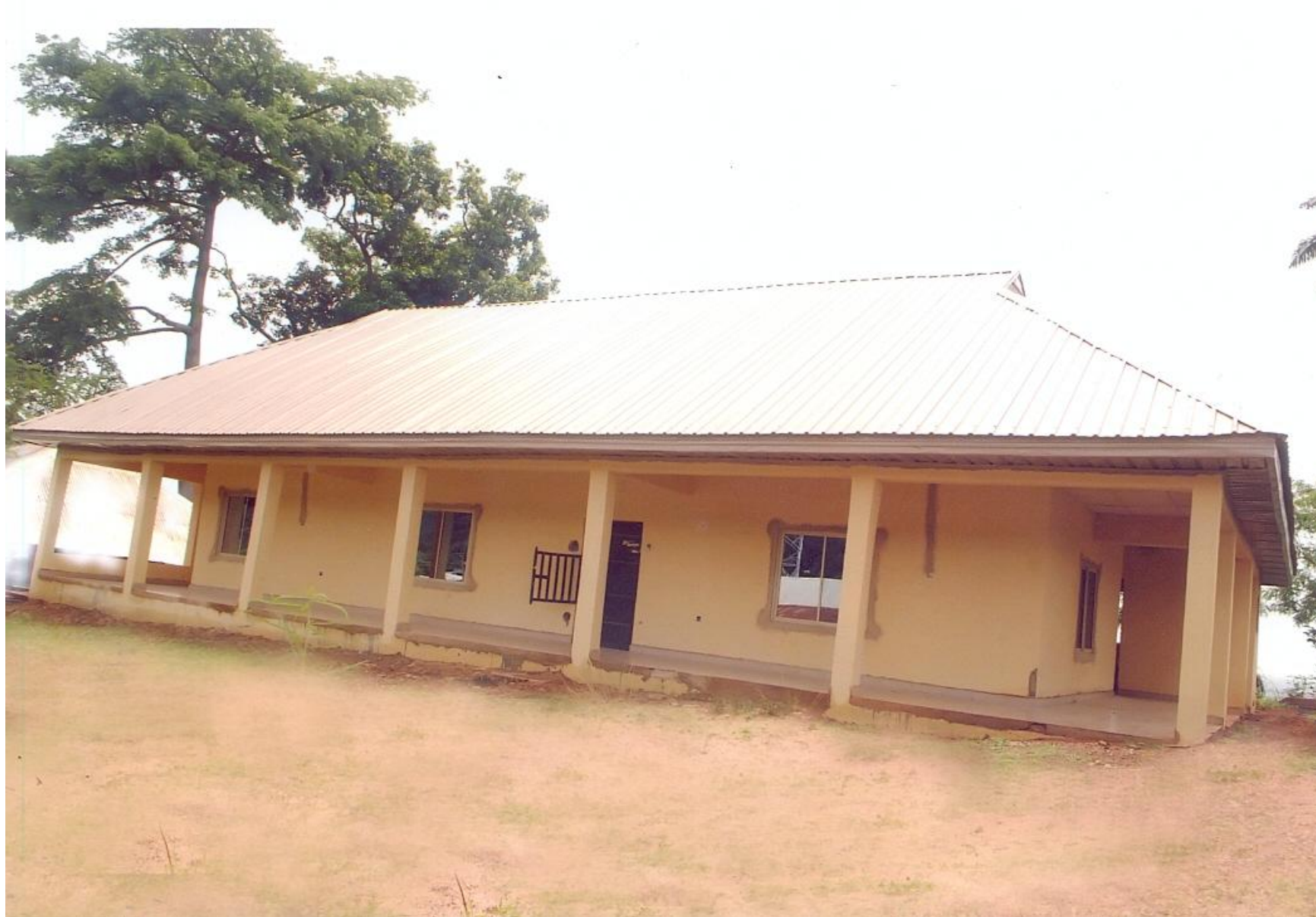
NEWLY RECONSTRUCTED AWGU SUB-TREASURY
