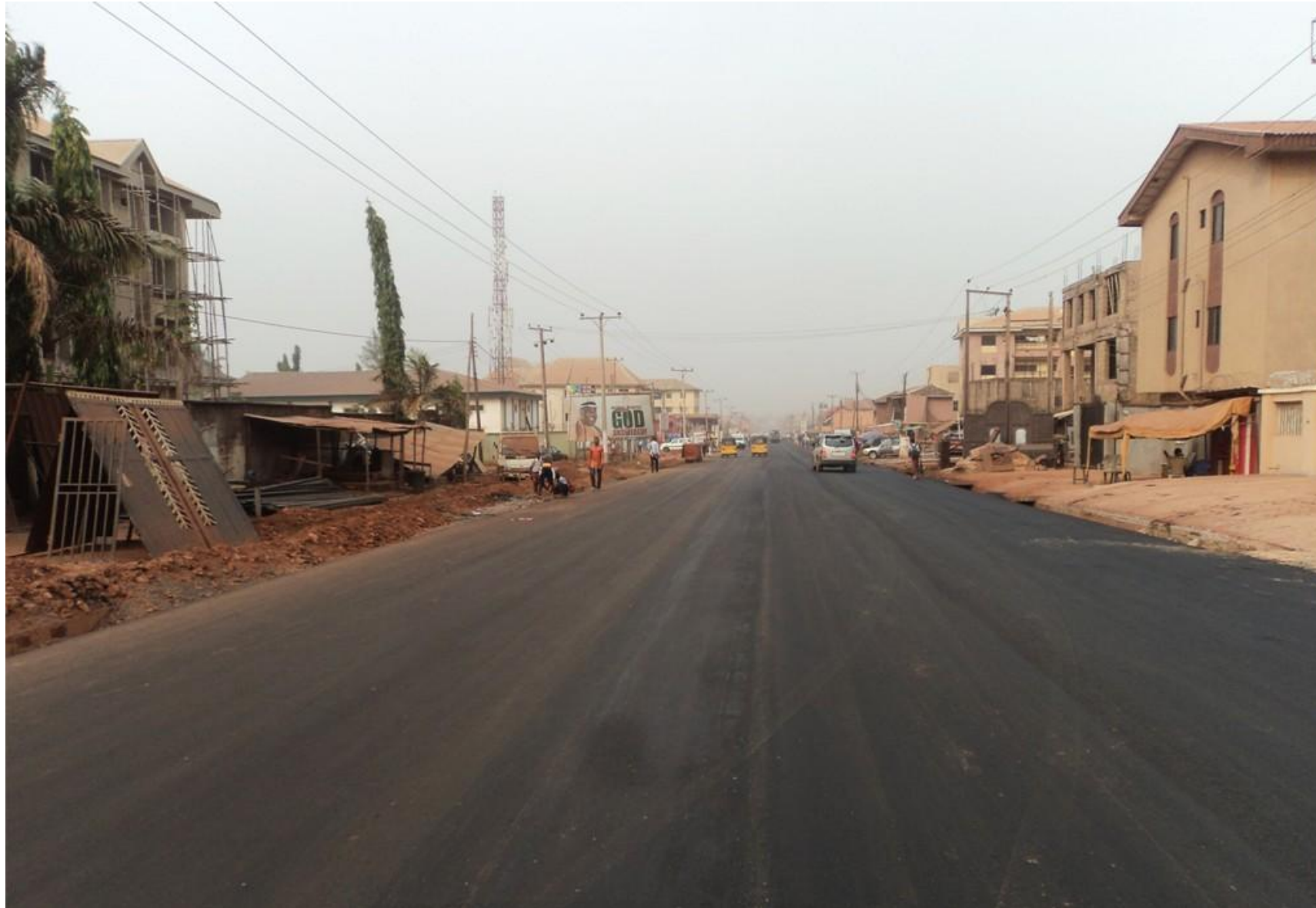
NIKE LAKE ROAD IN ENUGU EAST LOCAL GOVERNMENT AREA
